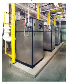
Futera boilers feature full modulation and 3:1 turndown, and are designed to supply the precise amount of heat necessary to maintain desired building temperature by matching heating demand without overfiring and wasting energy. A gasket-free heat exchanger with bronze headers and fittings prevents rust and corrosion for the life of the boiler. Finned tubes are industrial-grade copper with fins and tube walls formed as one for maximumheat transfer.
